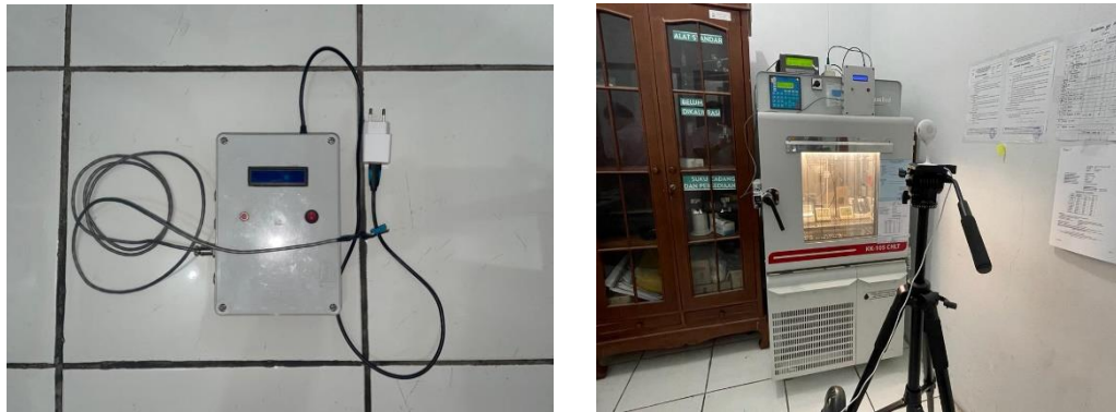
Figure 3. Overall view of the system after installation and assembly
